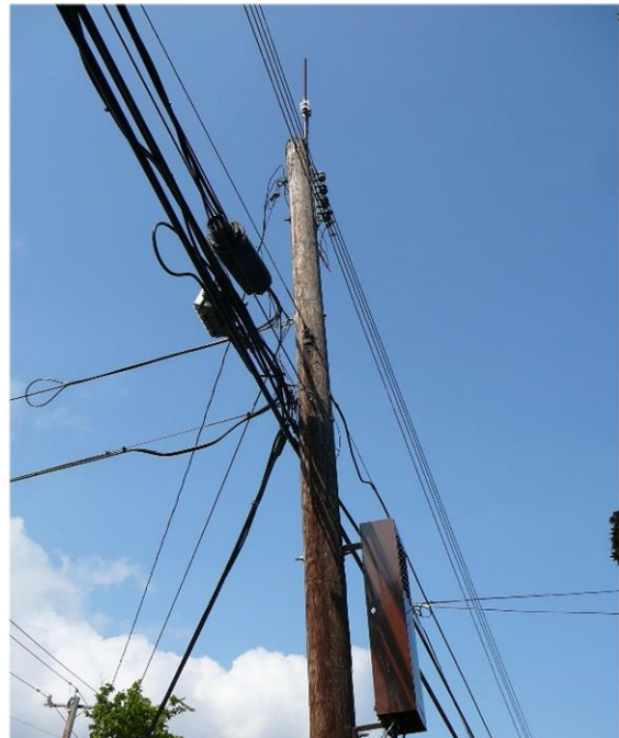
Figure 1 - An example of an electric pole with multiple telecommunication connections. https://upload.wikimedia.org/wikipedia/commons/4/47/NextGDAS.JPG
