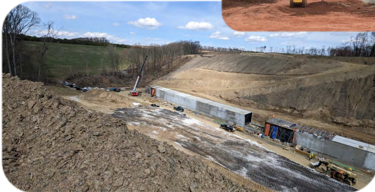
Stream Culvert Construction Downstream of Northern Ash Basin
