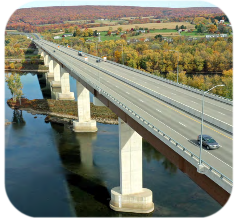
CSVT River Bridge (looking northeast)
