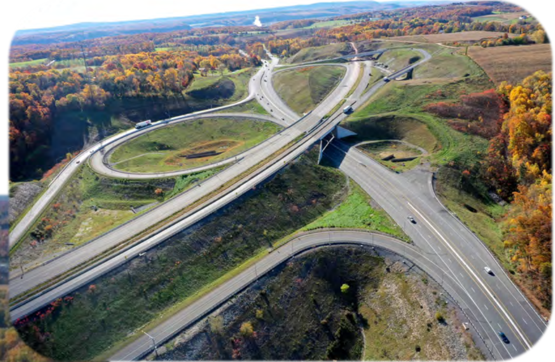
CSVT Interchange with US 15 (looking south)
