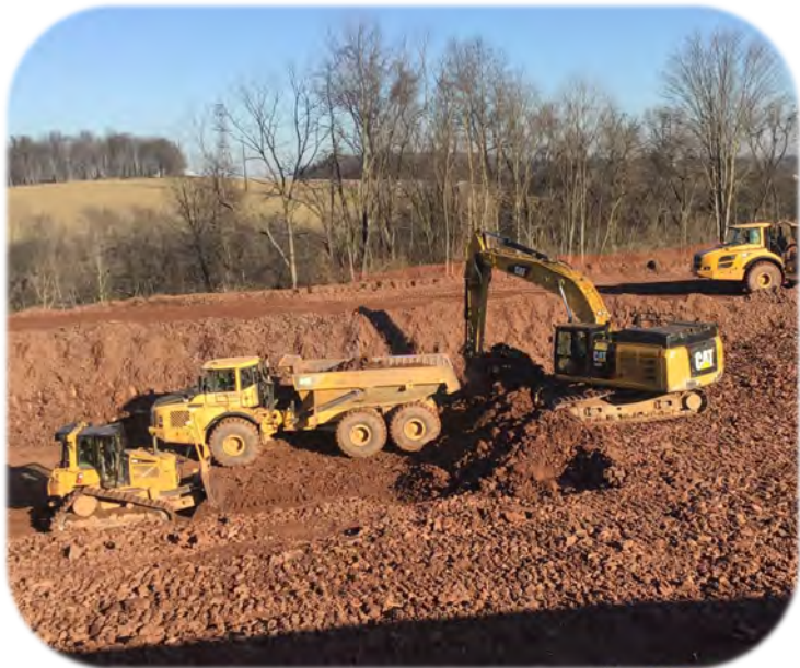
CSVT Excavation near Grangers Road
