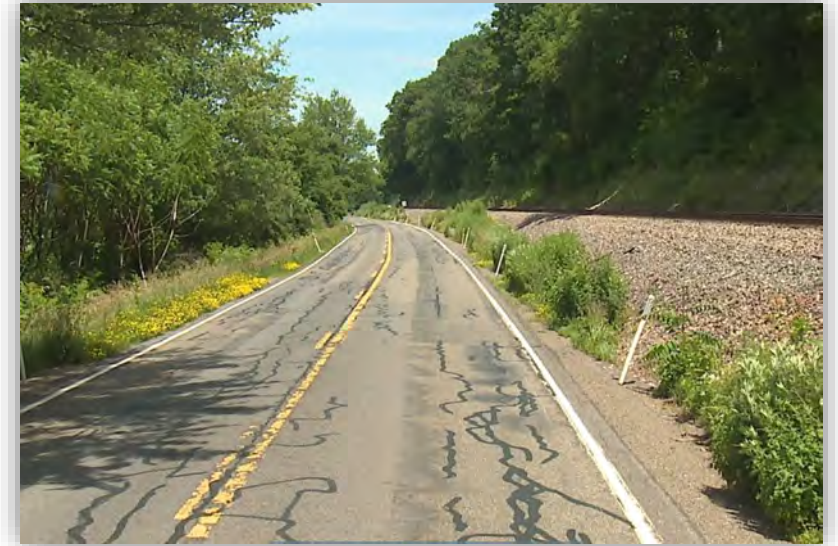
SR 339 in Mifflin Township Before
