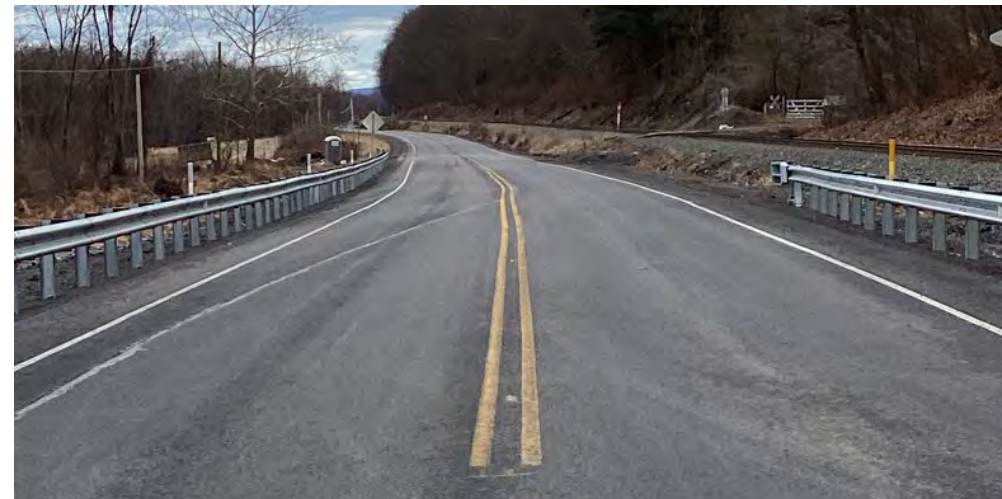
SR 339 in Mifflin Township After
