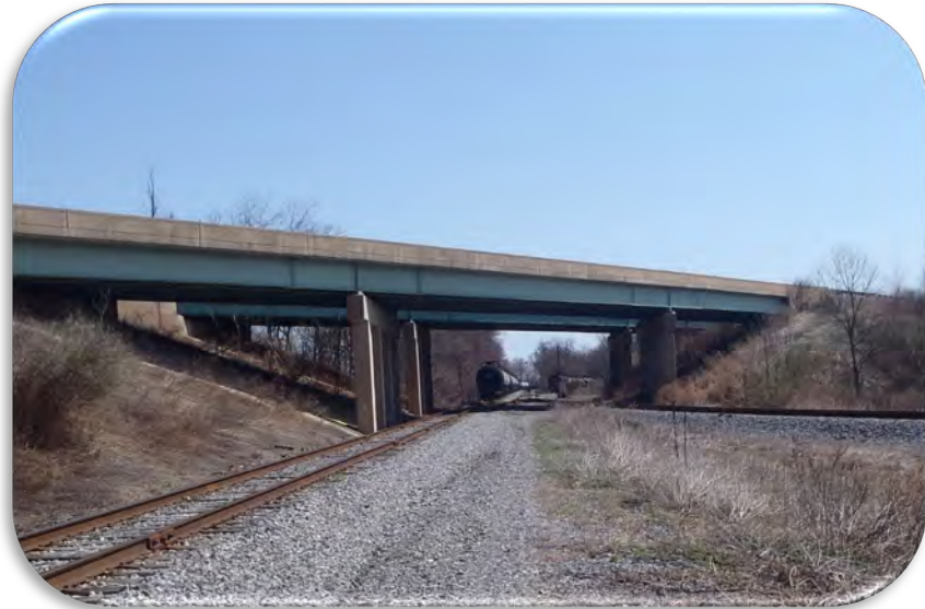
SR 220 over the Railroad Tracks
